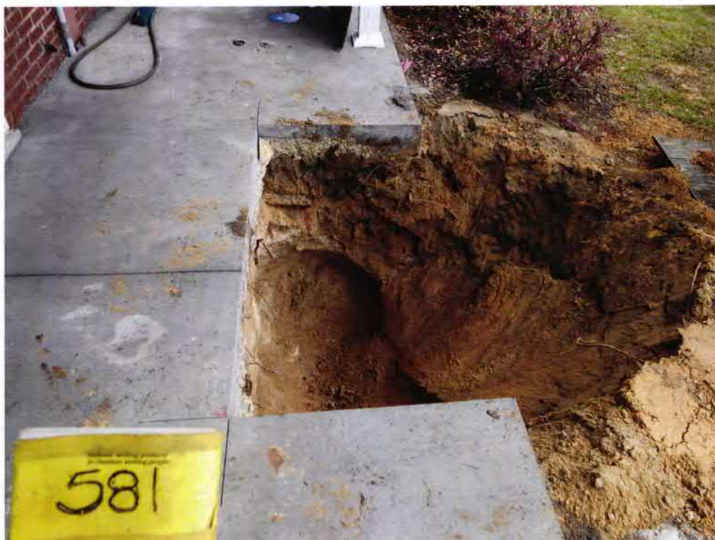
Picture 2: UST 581Aster excavation.
